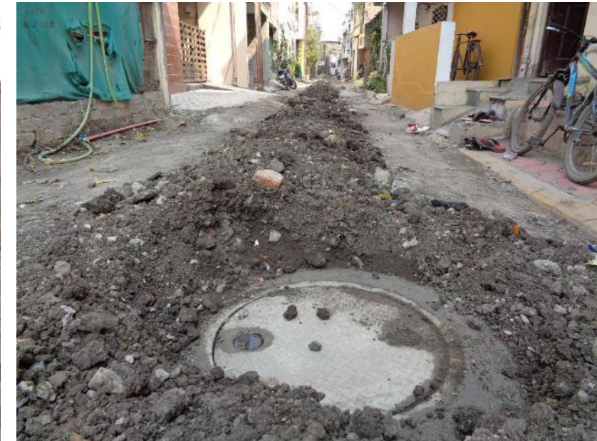
After sewerage system was installed and man-holes covered
